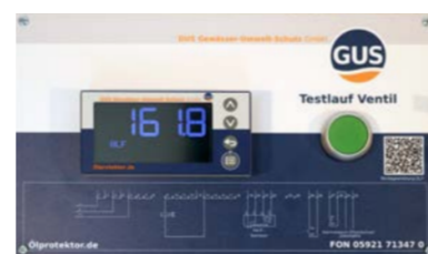
Switch box (control module) IP65-protected and UV-resistant
